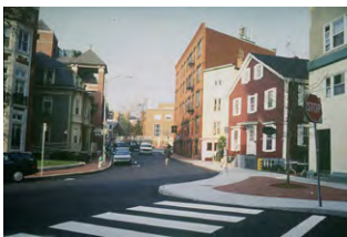
Traffic calming elements include raised crosswalks, special crosswalk paving materials and corner bump outs.
