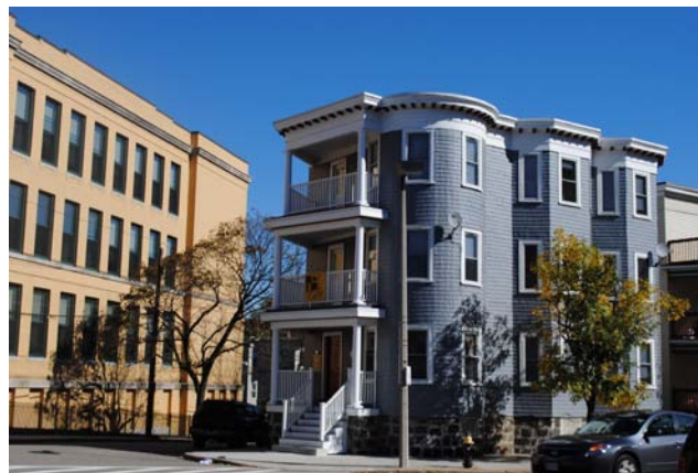
412 Talbot Ave, Post Renovation
